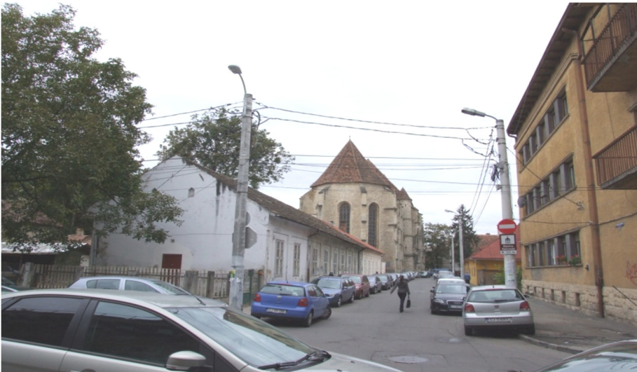
Fig. 2. Mihail Kogălniceanu Street view from the fortress wall, facing the Reformed church
